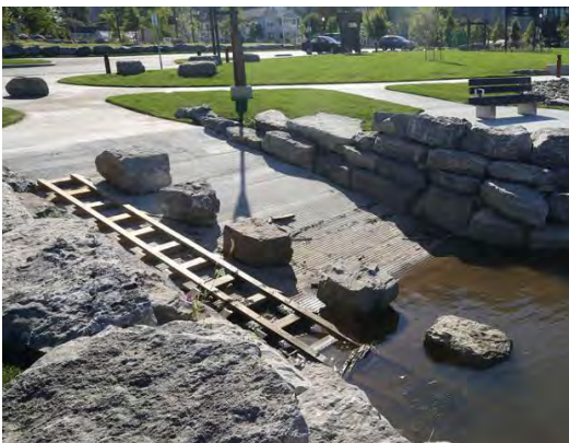
▲ Newly Renovated NYSDEC Boat Launch in Buffalo, NY; Image Credit: BuffaloBlueway.com
