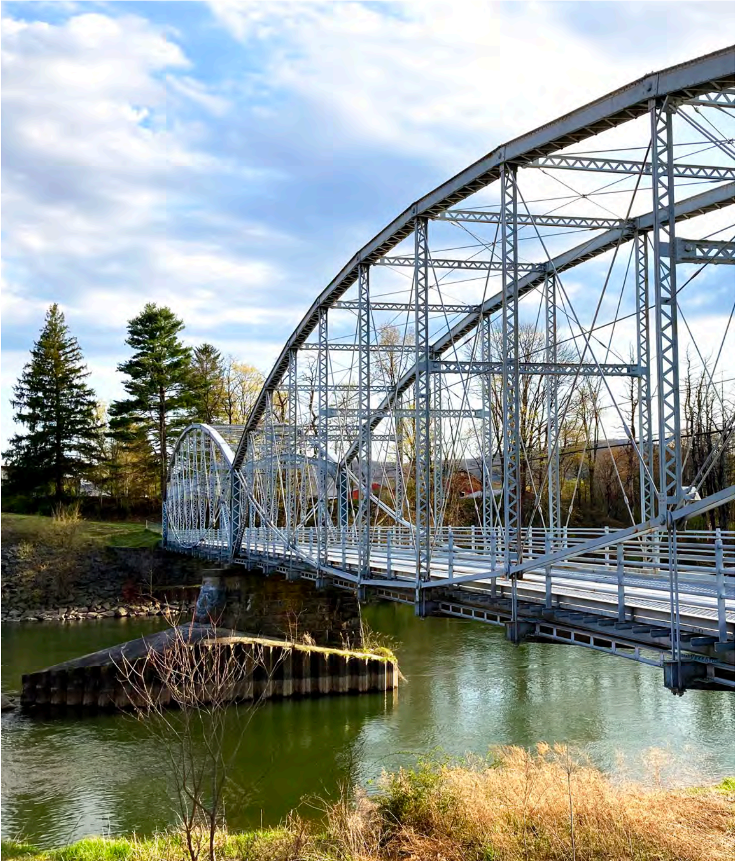
▲ Ouaquaga Bridge - Nearby Existing Major Water Access
