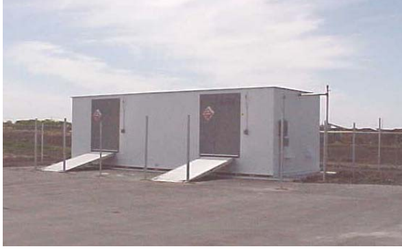
Figure 7-2. Hazardous Materials Storage Locker
