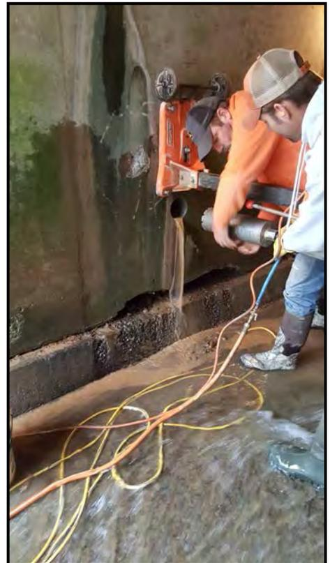
**Photo #3:** BIN 3360370 Stratmill Road Bridge – drilling weep holes in the abutment – Summer 2018.
