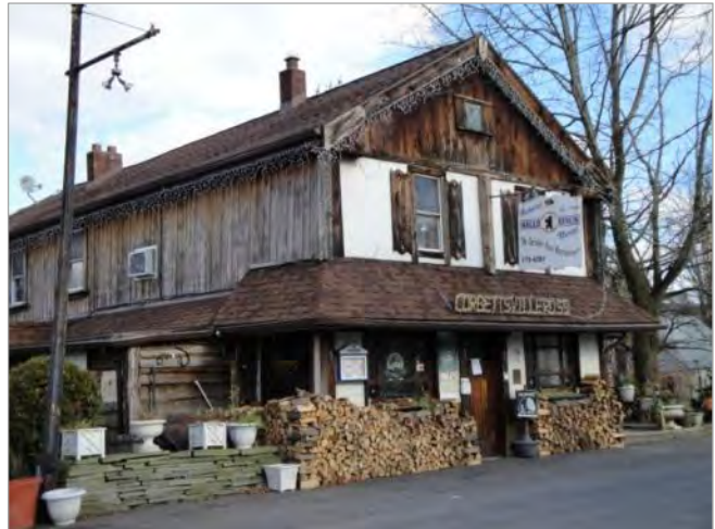
An extant commercial structure in the Hamlet of Corbettsville showcases the history still present in the Town of Conklin.
