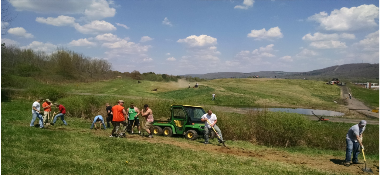
Constructing running paths, spreading crushed asphalt and mowing
