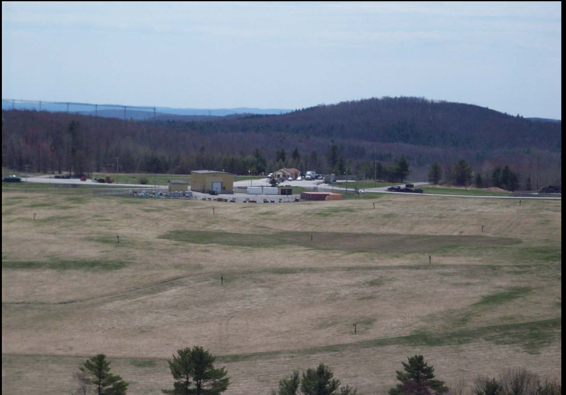
View of hazardous waste facility and scalehouse.
