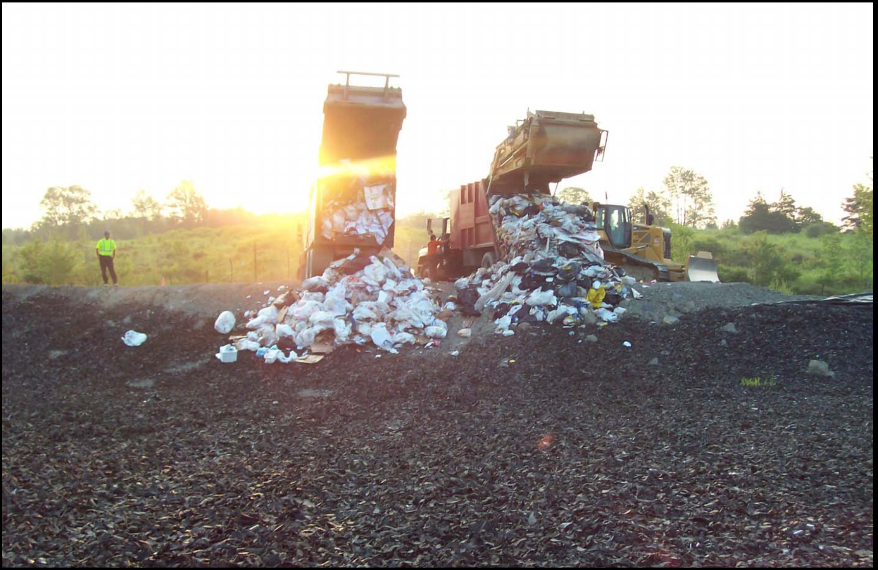
The first loads of waste are placed in Section IV Cell 1 of the landfill in August of 2009.
