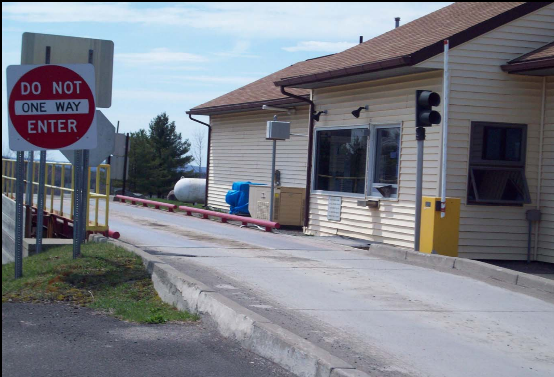
The inbound scales where vehicles weigh in & out. All vehicles must go over the scales.
