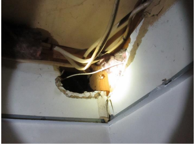
Ceiling where Meth was located
